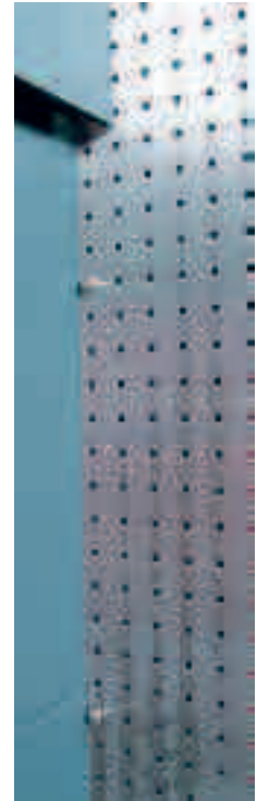
Figure 11: To prevent galvanic corrosion, only stainless steel fasteners should be used on stainless steel panels.
