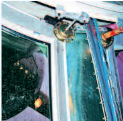
Figure 20: To prevent galvanic corrosion, the stainless steel cladding is fastened to the carbon steel inner structure in non-humid areas.
