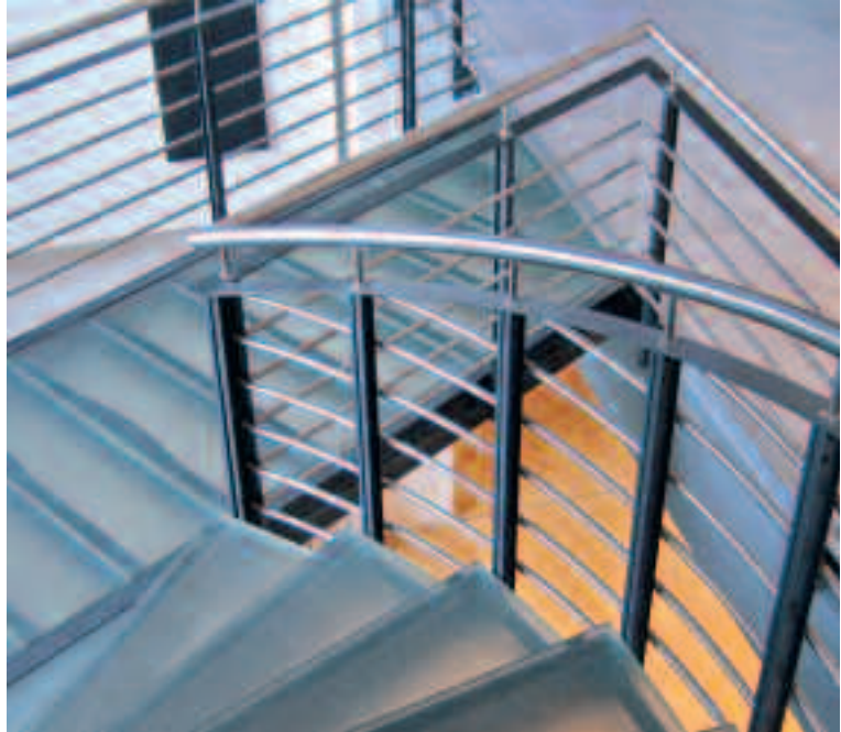
Figure 5: As electrolytes are typically absent in normally heated and aerated interior environments, the combination of stainless steel with other metallic materials such as painted carbon steel does not typically involve a risk of galvanic corrosion in such circumstances.
