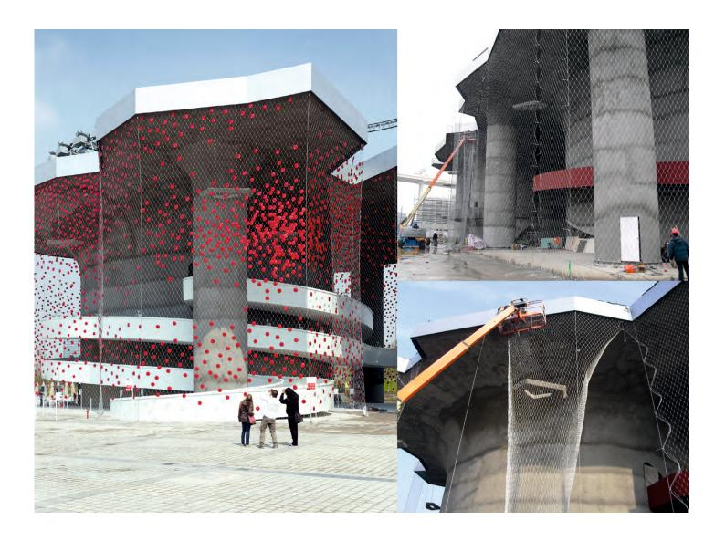
Several mesh stripes can be fixed together without any visible seam. This allows an easy installation of huge areas. After assembly of the stainless steel mesh, the LED-DOTS can be fixed with a stainless steel clamp by hand.
